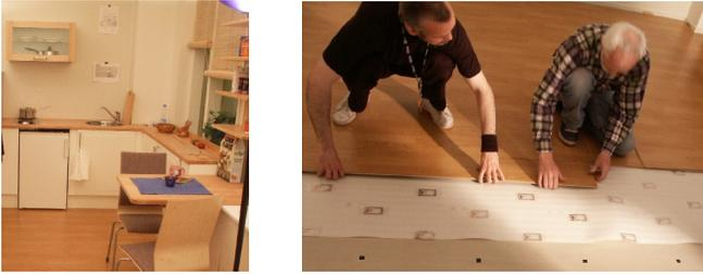
Fig. 4. The PEIS Home physical test-bed. Left: the kitchen. Right: the construction of the floor, showing the grid of RFID tags.
